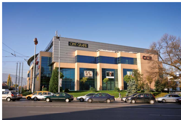
City Center Sofia, Bulgaria – Interior lighting ESTRELLA Series, PROFFIT Series
