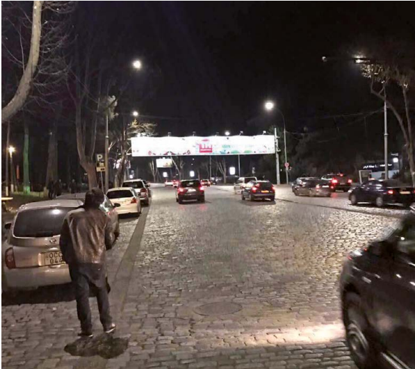
Tbilisi Municipality, Georgia – Street LED lighting EXTREME UHE Series
