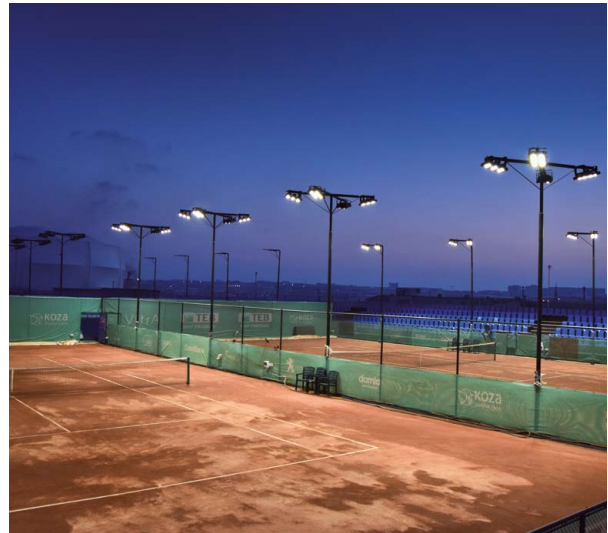
Garanti Koza Tennis Complex, Istanbul, Turkey – Training outdoor and indoor courts, MEGA Series
