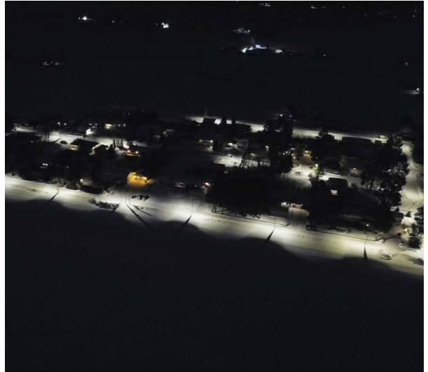
Elin Pelin, Sofia District- Smart Street Lighting EXTREME FLAT UHE Series
